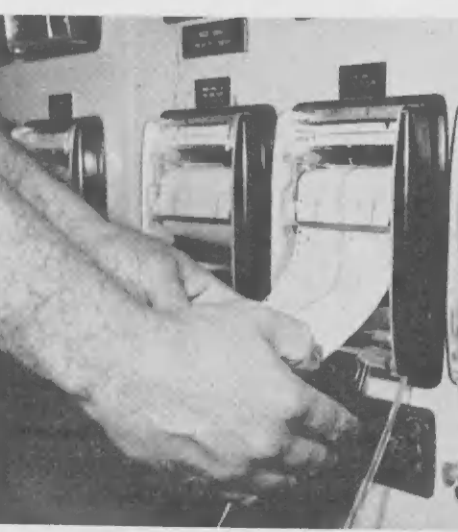
-ROUGHPUT is continuously and accurately recorded on delicate flow o recorder control instruments installed in unit control houses. ACION di Lago ta worde continuamente y exactamente registrá ariba in- strumentonan delicado den control house di e plantanan.
